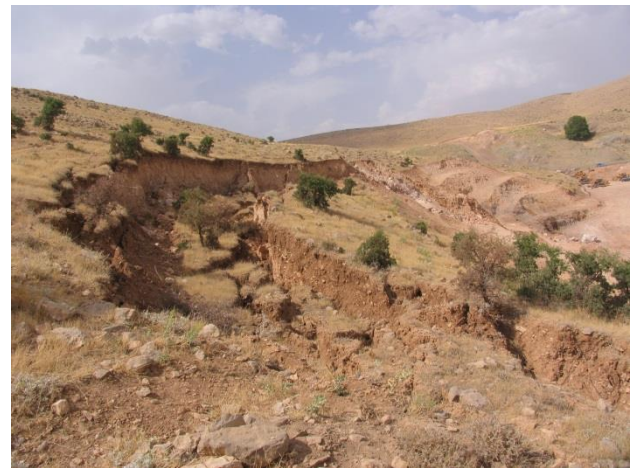
Figure 13. The head scarp after removing the landslide's toe
