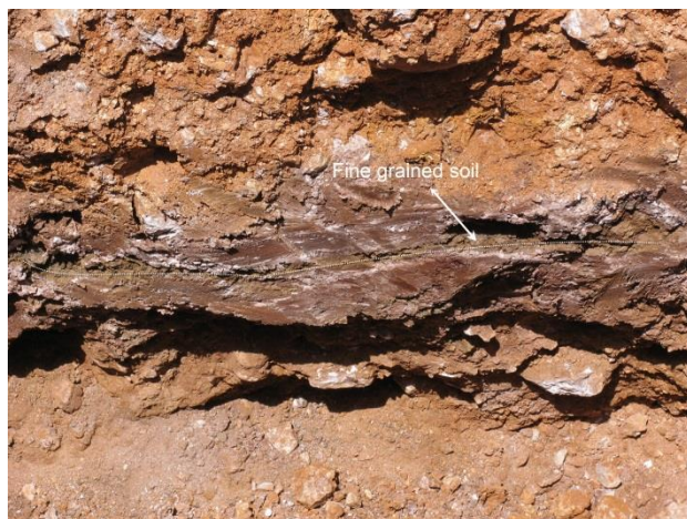
Figure 8. The discrete shear zone of the ancient land slide in the trench opened on the R.O.W
