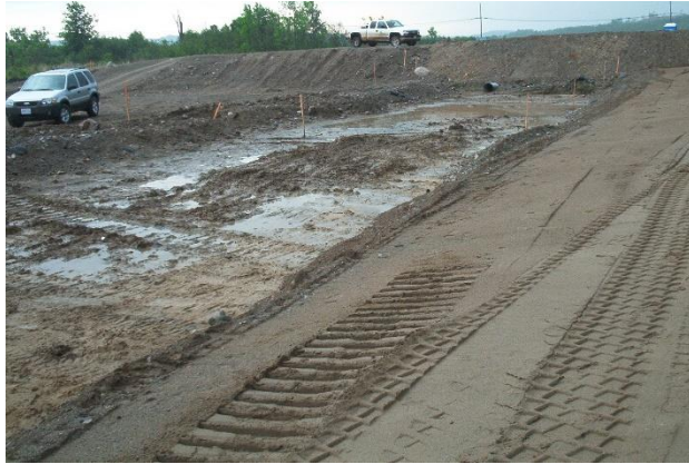
Figure 6 – Highway 17 construction (2005) – culvert embankment in background
