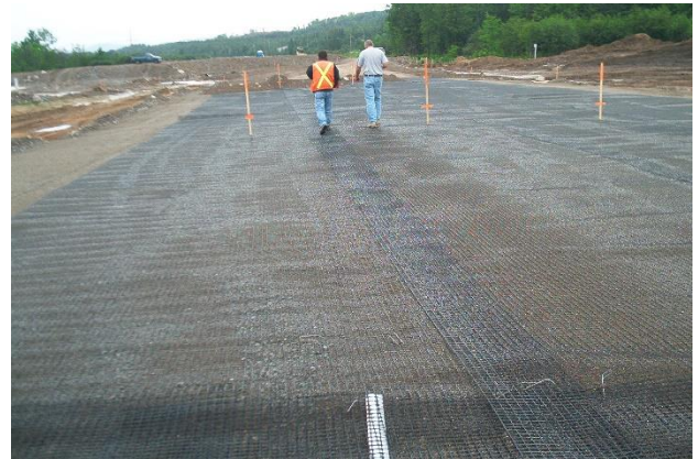
Figure 18 – June 14, 2005 – Embankment Reconstruction
