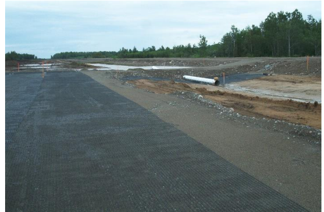
Figure 17 – June 14, 2005 – Embankment Reconstruction
