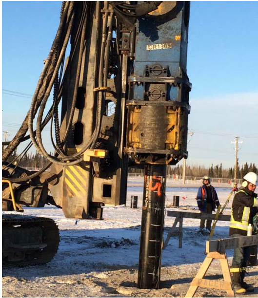
Figure 8. PDA Testing Set Up.
