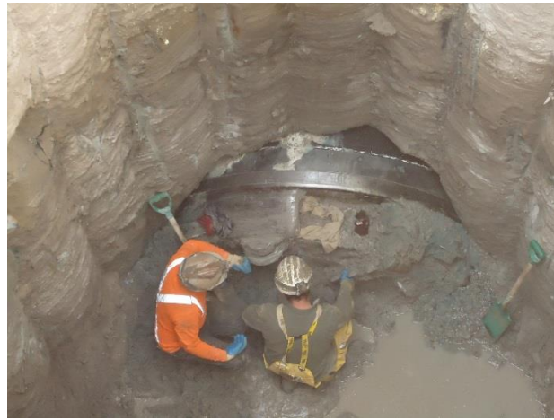
Figure 1. View of TBM within rescue shaft
