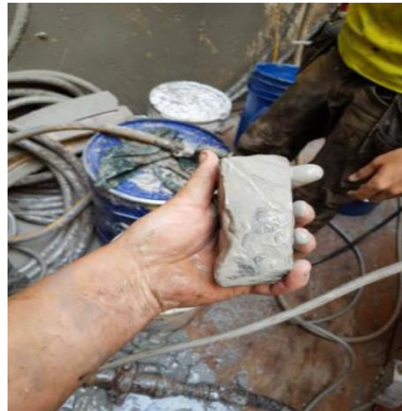
Figure 3. View of cut rock fragments removed from MTBM slurry return lines
