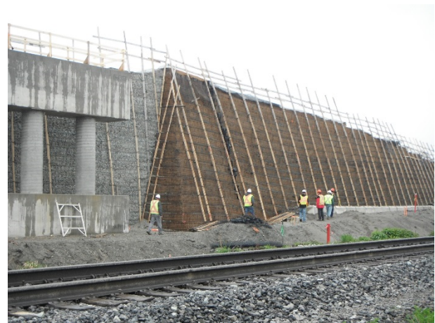
Figure 10. Photograph showing the partially completed L760 embankment
