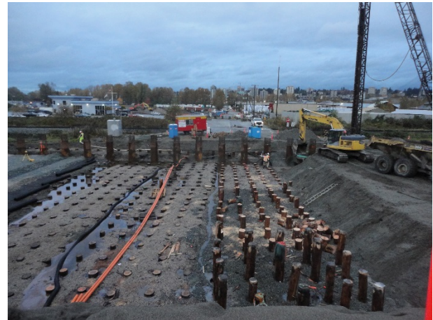
Figure 9. Photograph showing installation of the timber piles
