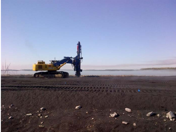
Figure 2: Photo of Rapid Impact Compaction Rig in Operation
