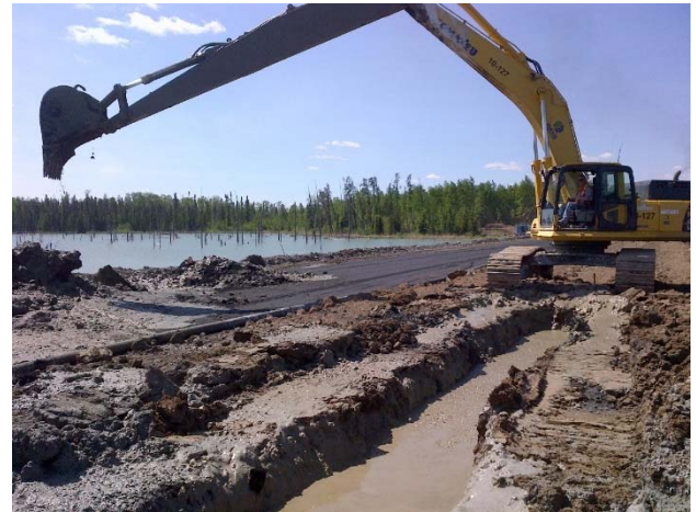
Figure 5: Photo of long reach excavator on site
