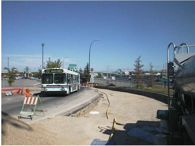
Figure 6. Excavation prior to July 22, 2000 placement of cellular concrete
