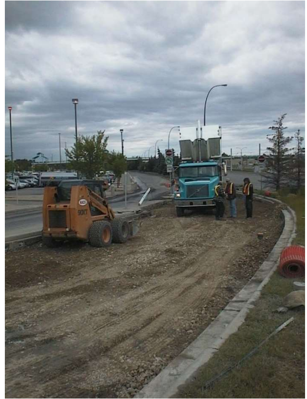
Figure 10. Photo taken during gravel placement.
