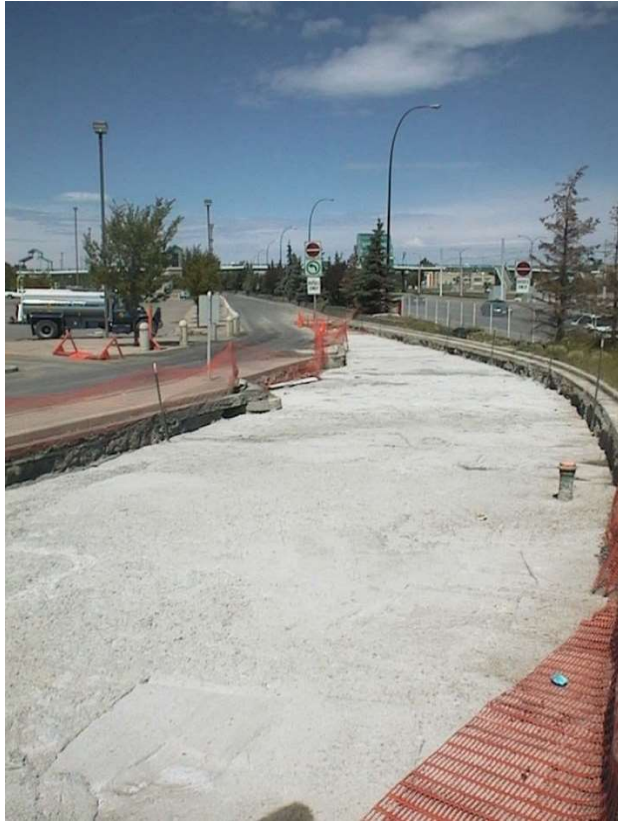
Figure 9. Photo taken after placement of LCC.
