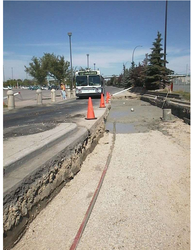
Figure 8. Photo taken during placement of cellular concrete.
