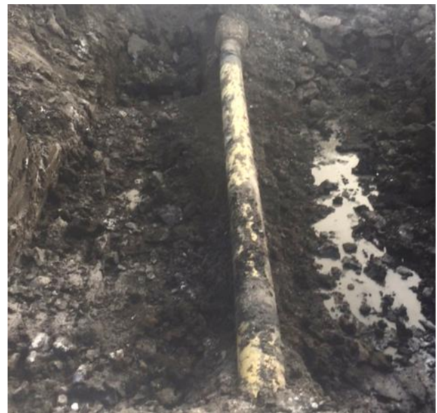
Figure 3. Horizontal Displacement of the Pipe
