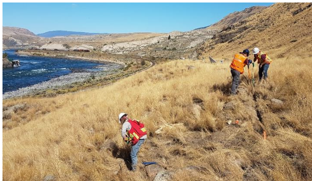
Figure 3. Installation of ERT system
