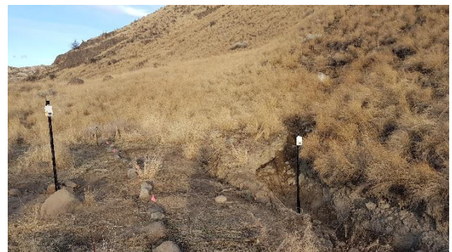
Figure 4. Matric suction instrumentation relative locations on the landslide an in the head-scarp
