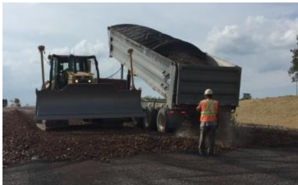
Figure 1. Placement of the aggregate on the geogrid
