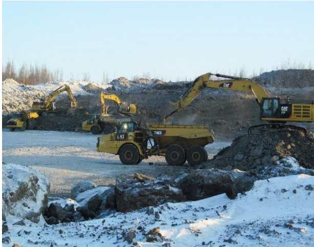
Figure 4. Winter construction activities in borrow source.
