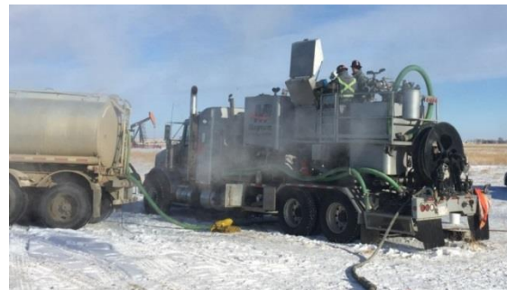
Figure 4: Pumping & placement of pill
