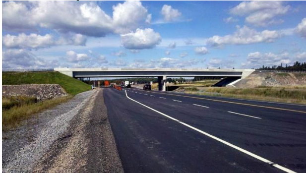
Figure 6 - Looking North at Underpass after Completion
