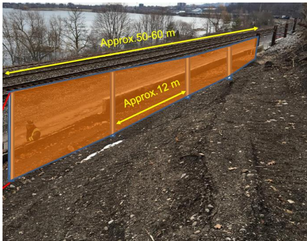
Figure 10. Proposed rockfall barrier extension viewed downslope
