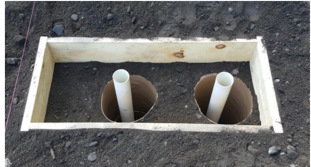
Figure 10. 12" sonotubes, 8" thick concrete pad and 3" PVC sleeves
