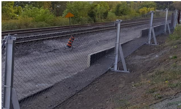
Figure 13. Rigid post barrier extension viewing downslope
