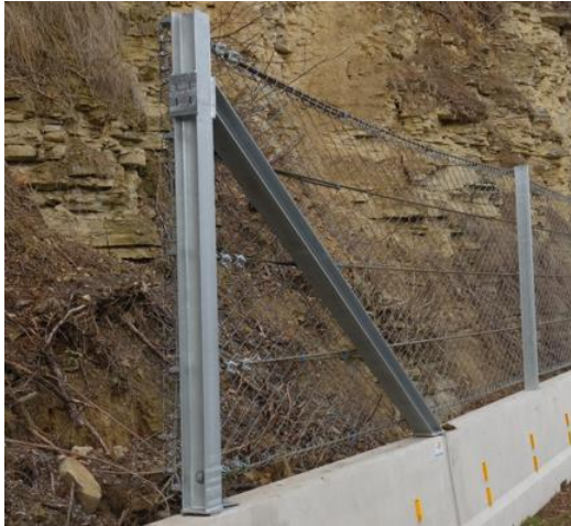
Figure 4. Rigid end post of a Geobrugg rockfall barrier braced by a compression member
