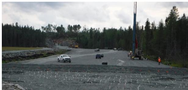
Figure 2. Wick drain installation at Station 14+650
