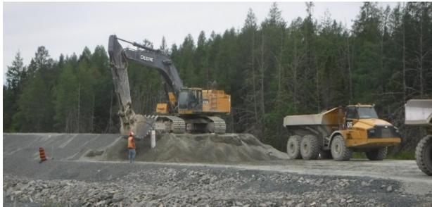
Figure 4. Removal of granular surcharge material
