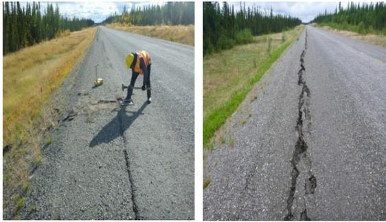
Figure 4. Pronounced edge cracking at KM 66.275 in spring 2017 (right), as a comparison to spring 2016 (left)
