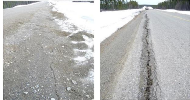
Figure 3. Edge cracking at sites 4 and 6 (left), and outside of site 6 (right) (from Bradley et al. 2017)
