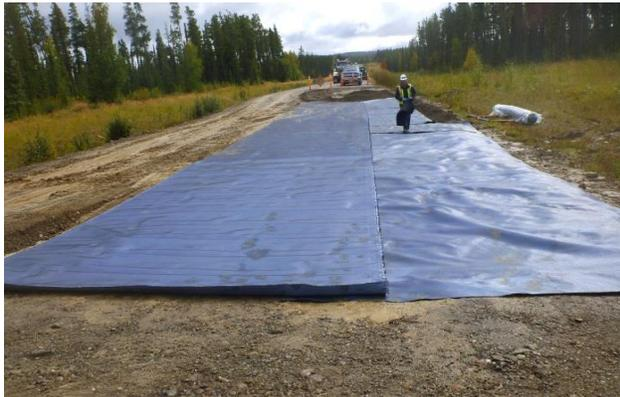
Figure 2. Wicking geotextile installation (Bradley et al. 2016)
