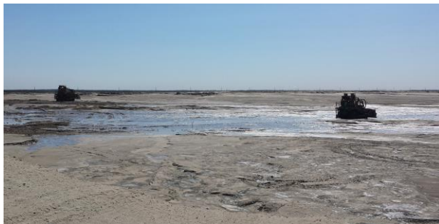
Figure 13. Dozers packing the SC2 beach during the wet beach trial.
