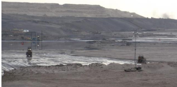
Figure 4. Track packing in the SEA in 2013.
