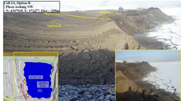
Figure 13: Pad ramp-down and safety berm
