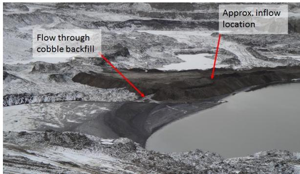
Figure 4. Erosion of initial backfill placement
