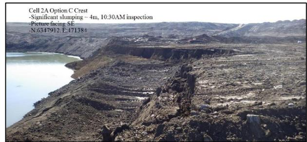
Figure 15. Slumping was typically preceded by cracking, and the slumping occurred slowly. Note the 4 m drop with significant extents. Photo from May 2015.
