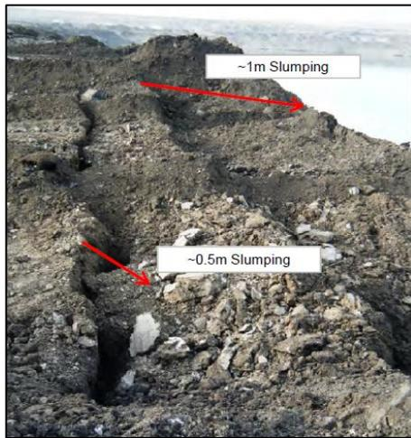
Figure 6. Pad slumping during construction – cracks observed ~ 2m behind the crest, August 2011
