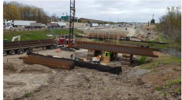
Figure 3a - Site #1 Pile Load Test Set-Up
