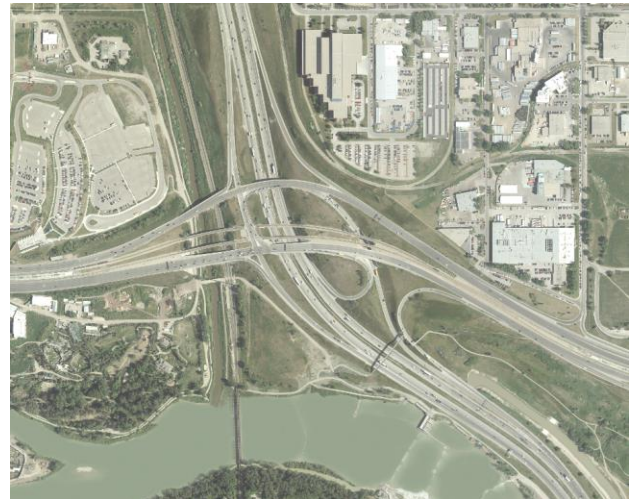
Figure 5. Deerfoot Trail and Memorial Drive Interchange located within 13-24-1-W5M.
