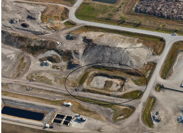
Figure 1. Area of Landfill Cell Construction.
