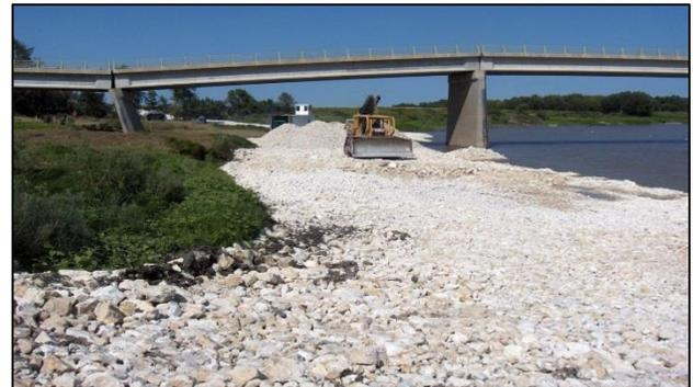
Figure 11. Construction of lower toe berm nearing completion under the bridge.
