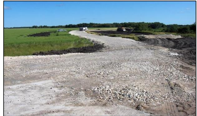
Figure 10. Construction access haul road, set back 20 m from top of bank and extending 70 m downstream from bridge.
