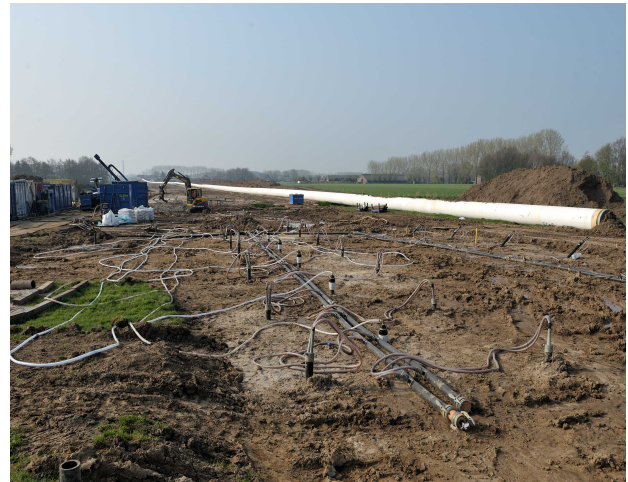
Figure 4. Bio-cementing of gravel for borehole stability field project (picture shared by van Paassen Leon).
