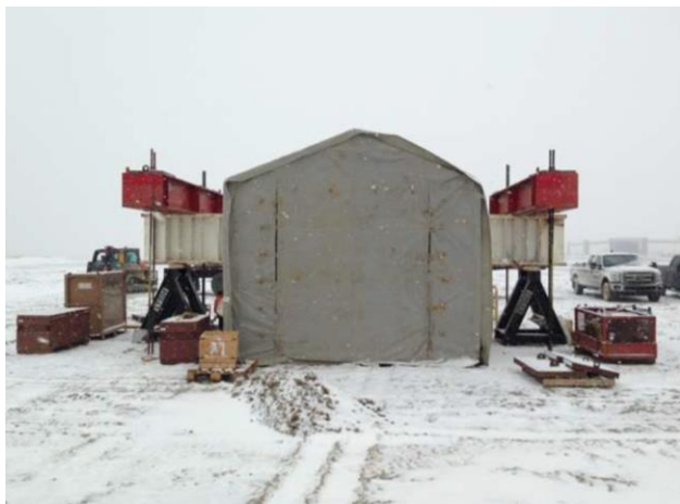
Figure 6: Pile load setup with four reaction piles
