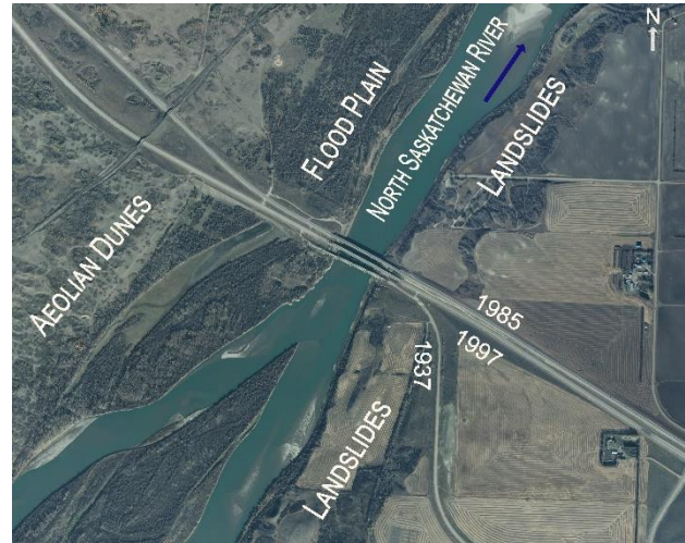
Figure 2. Aerial image of Borden Bridge site and landforms (after Panesar et al., 2014)
