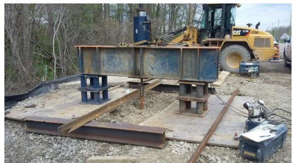
Figure 6- Sacrificial Rock Anchor Pull Test Configuration
