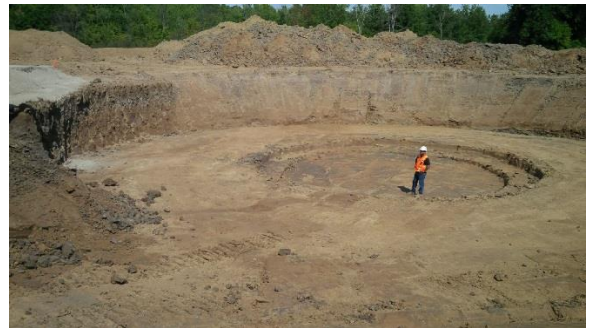
Figure 3- Competent Foundation Subgrade.
