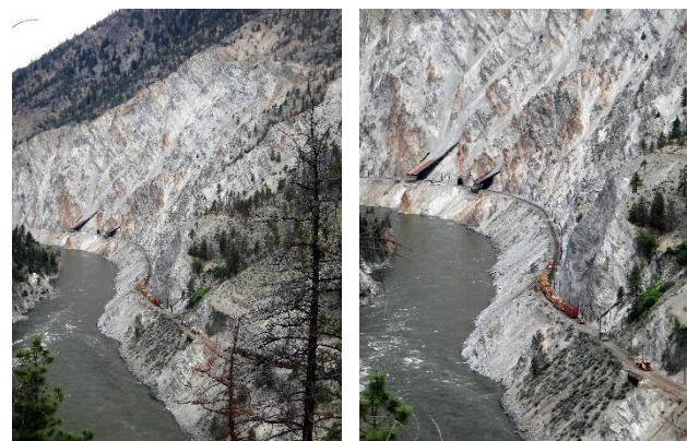
Figure 14: Ditch maintenance – White Canyon slopes.
