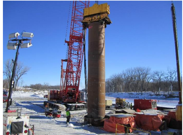
Figure 8: Advancing steel casing for rockfill columns at mid-bank.
