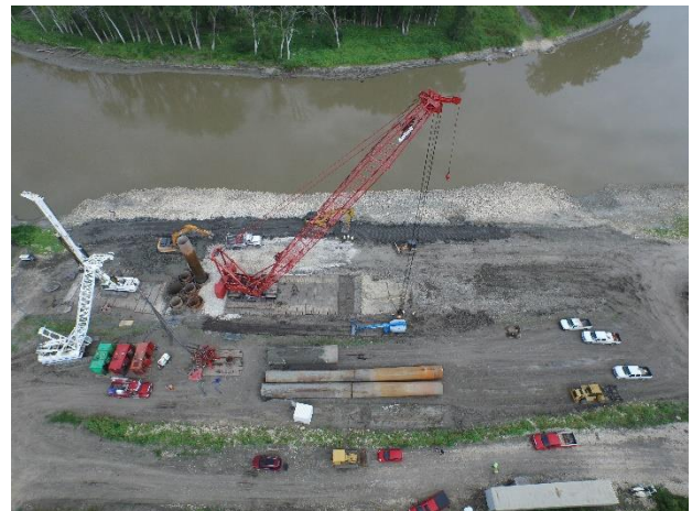
Figure 9: Installation of rockfill columns along mid-bank in August, 2015.
