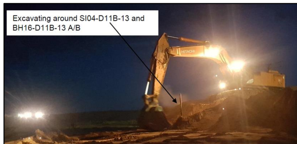
Figure 7. Excavation around the Instruments
