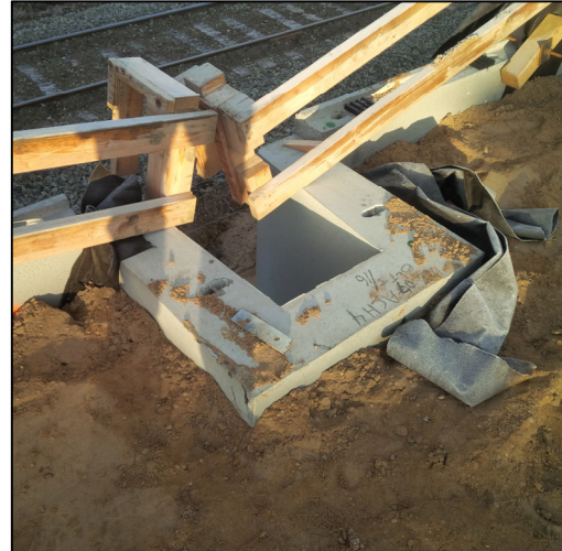
Figure 8. Drain Chase Element in Construction
