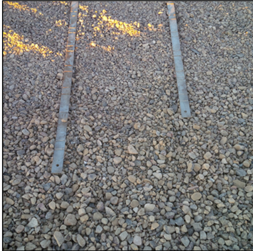
Figure 7. Soil Reinforcing Strips in Winter Backfill
