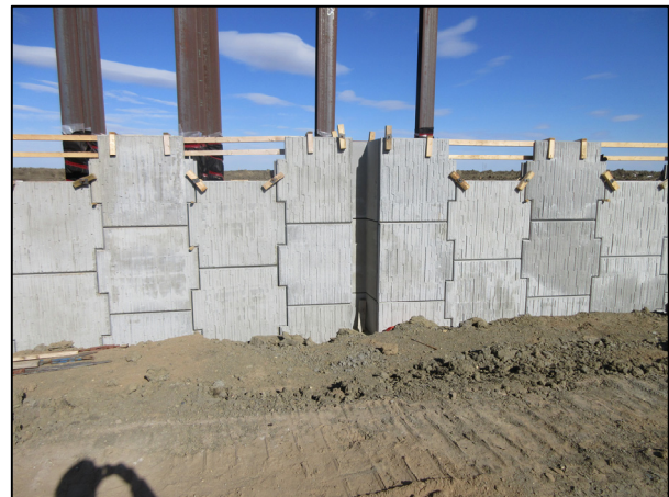
Figure 9. Drain Chase Element Installed in Wall S-RW-09
