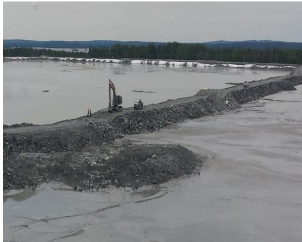
Figure 1. One of the waste rock inclusions in the tailings impoundment at the Canadian Malartic Mine (in 2017)
