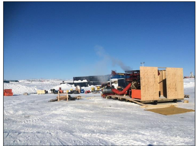
Figure 6. Drill Rig Assembly at the sealift beach in Iqaluit
