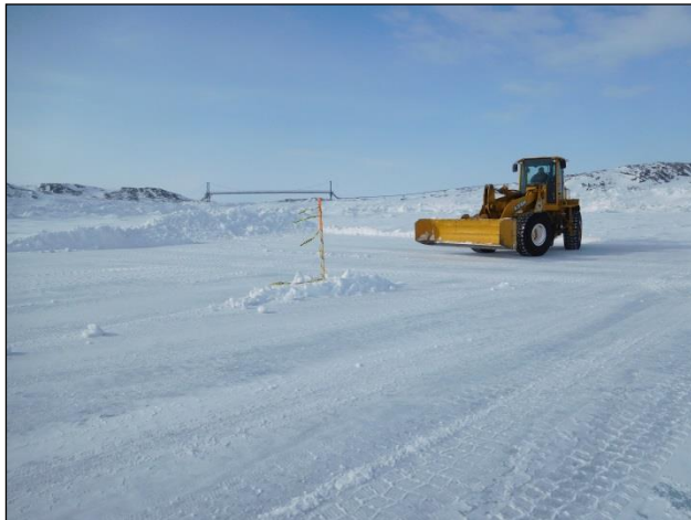
Figure 8. Road access and pad preparation
