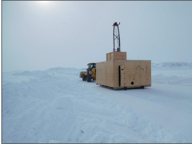
Figure 7. Assembled shack being towed to deep sea port area
