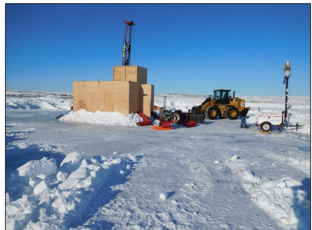
Figure 9. Typical drilling setup at borehole locations
