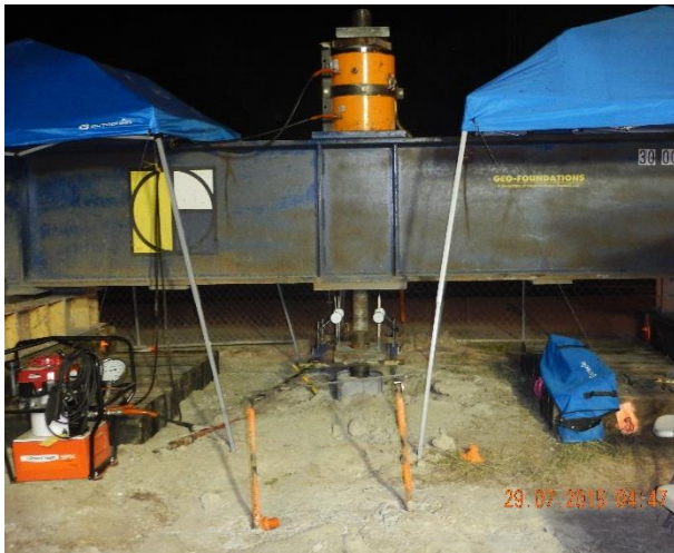
Figure 10. Load test arrangement
