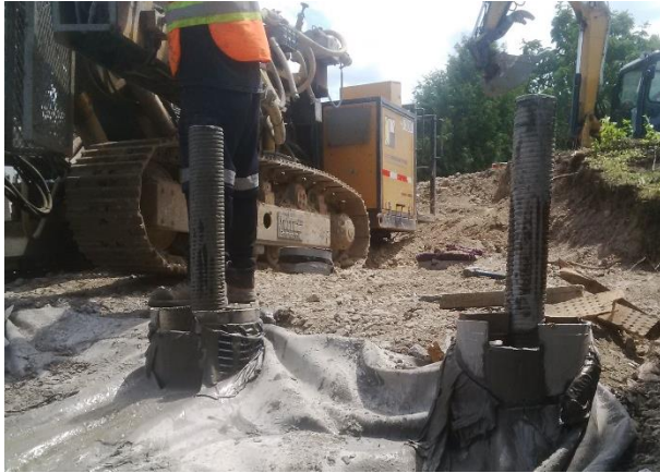
Figure 9. Two completed production micropiles
