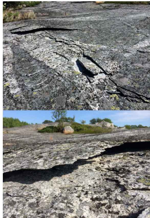
Figure 2. Observed fractures from the summer of 2014 (pictures courtesy of Mr. Sarpaneva).
