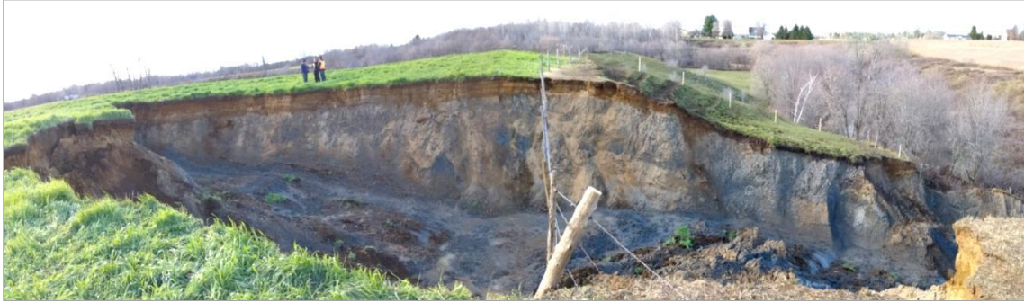
Figure 3. View of the scar of the first episode of flowslide, taken on November 9 th 2016, a few hours before the major event
