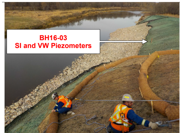
Figure 13. Final as-built remediated surface on November, 2016 (view looking north).
