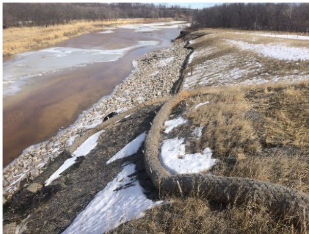
Figure 15. Final Remediated Surface 16 months after construction, March 2018 (view looking north).
