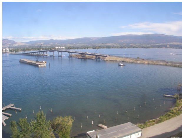
Figure 2. Photograph showing the bridge crossing
