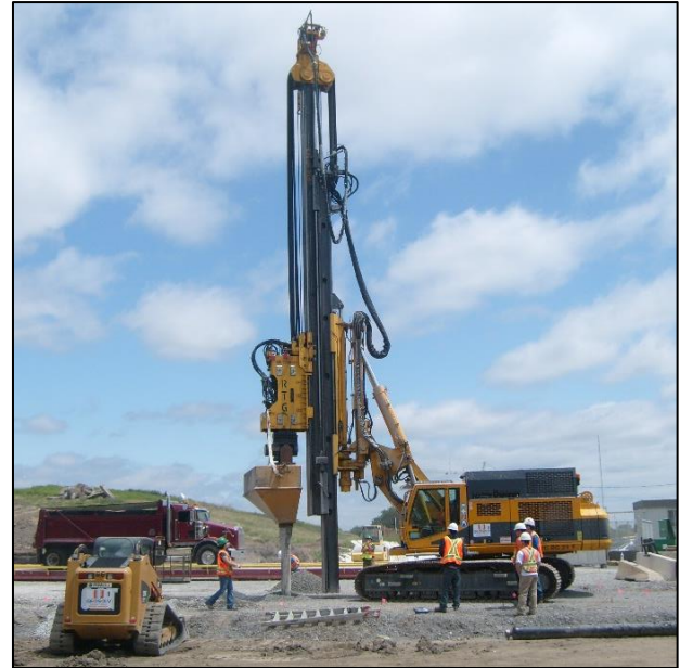
Figure 6. Photograph of the RAP installation.
