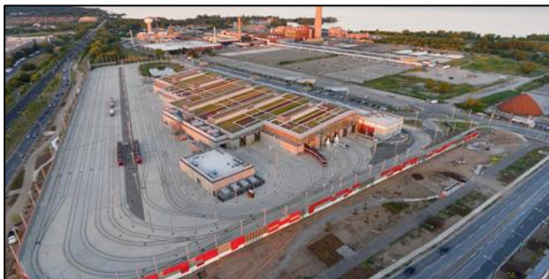
Figure 2. Photograph of completed facility.
