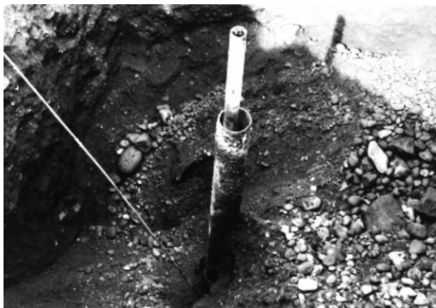
Figure 6 Survey "benchmark tube"
