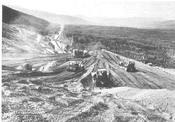
Figure 2 South Moraine – bulldozer loading the hoppers which feed the conveyors
