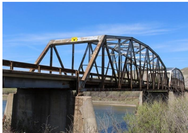
Figure 2. Existing bridge configuration looking from west to east
