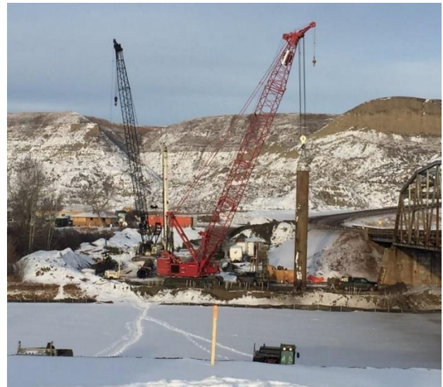
Figure 6. Typical cast-in-place pile installation setup
