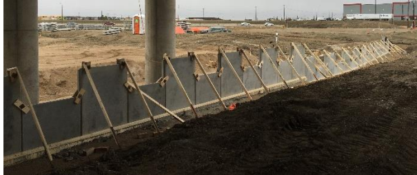
Figure 16 – First Row of Panels Installed
