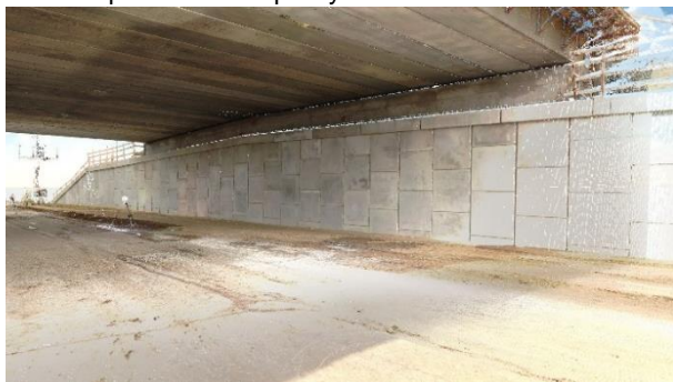
Figure 3 – Project Point Cloud of North Wall on August 28
