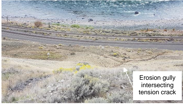
Figure 5. Flow path directed into landslide head scarp
