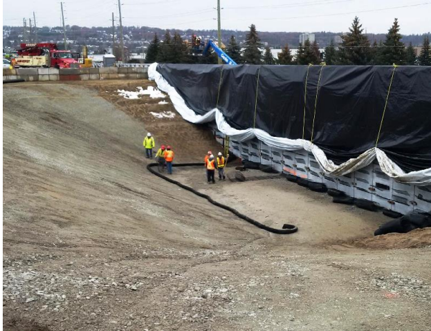
Figure 14. Excavation prepared for LCC placement
