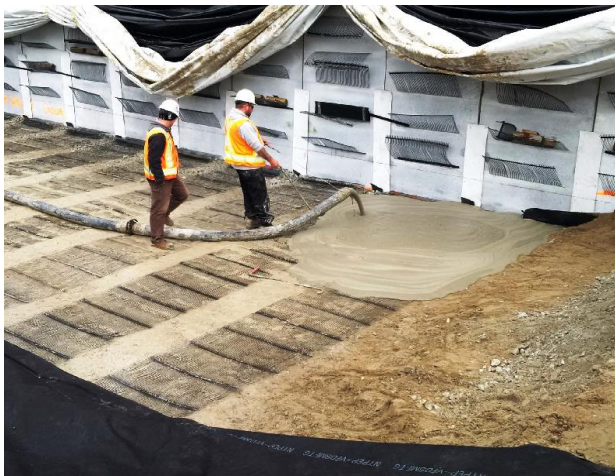
Figure 15. LCC pouring over geogrid reinforcement in progress
