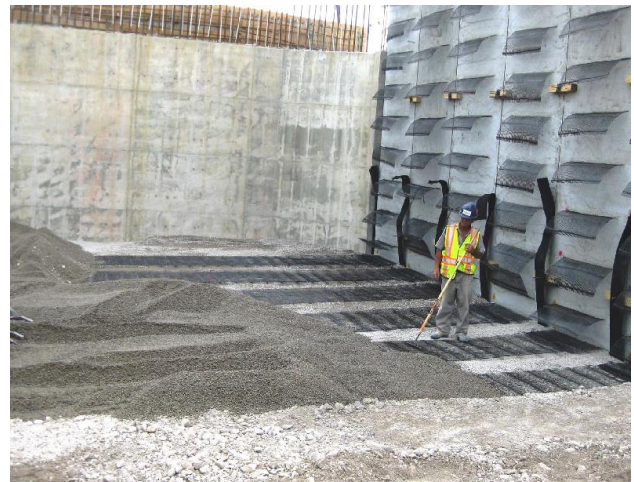
Figure 10. FS placement behind the MSE wall
