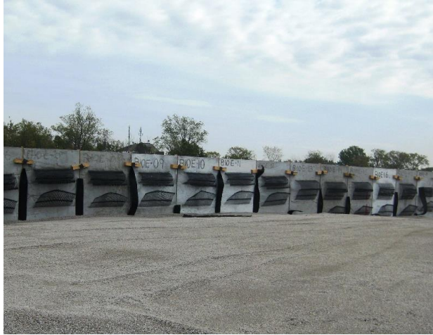
Figure 11. FS backfill near the top of the MSE wall
