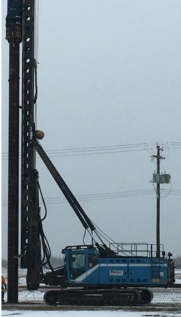
Figure 1. Typical Onshore Pile Installation Set-up
