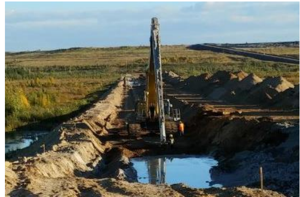
Figure 2. Excavation of the COW under slurry
