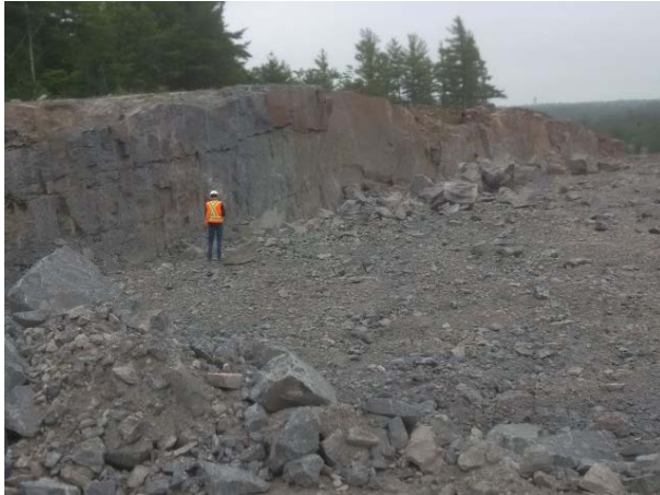
Figure 2. Bedrock cut along future highway at borrow source of Ojibway.
