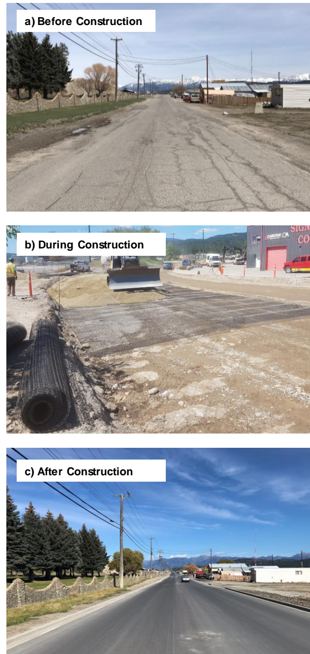
Figure 2. Before and After Rehabilitation of Cobham Ave West
