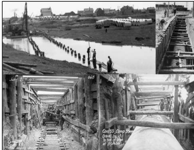
Figure 1: Original Construction of Branch 1 Aqueduct.
