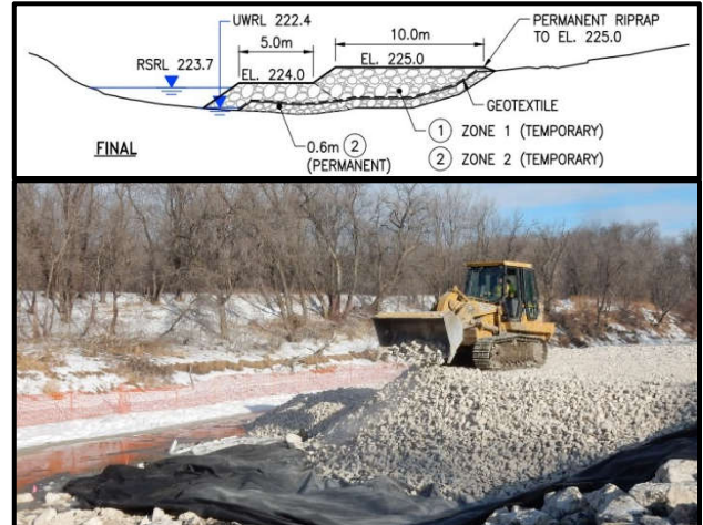
Figure 4: Permanent Riprap Blanket and Temporary Rockfill Berm.
