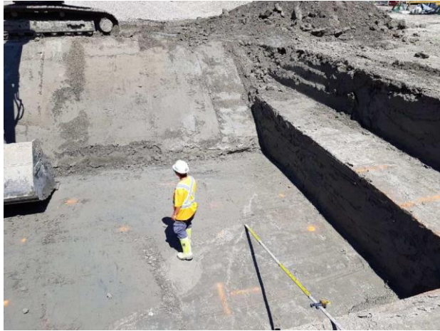
Figure 8. Foundation pad with sloped wall after removal of weak soil zone
