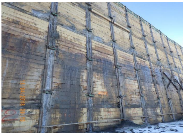
Figure 6. Completed temporary shoring system
