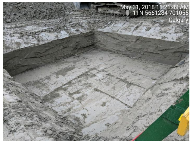
Figure 7. Typical foundation pad cut within till
