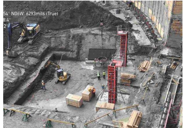
Figure 12. Completion of Tower Crane 1 footing (facing west)
