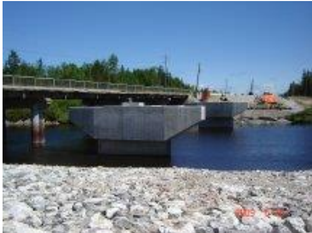
Figure 1. Kabinakanagi River Bridge (facing east)
