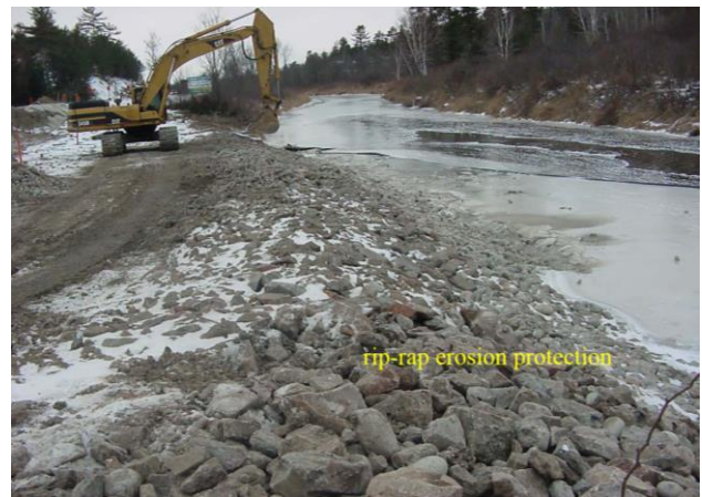
Photo 6. Rip-rap erosion protection in the river channel
