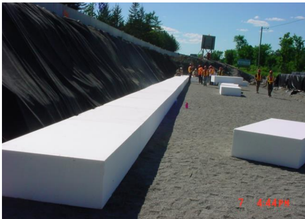
Photo 5. EPS fill placement
