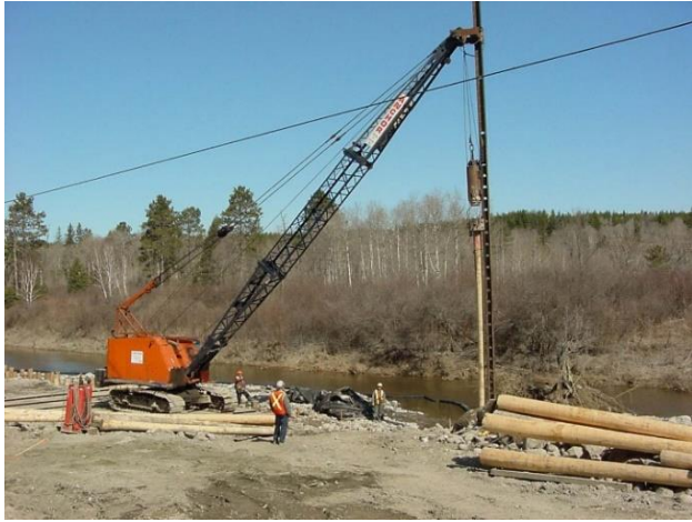
Photo 4. Timber pile installation
