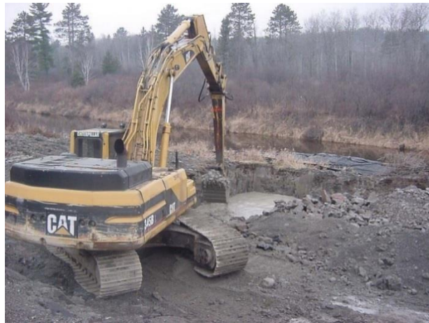
Photo 2. Shear key construction
